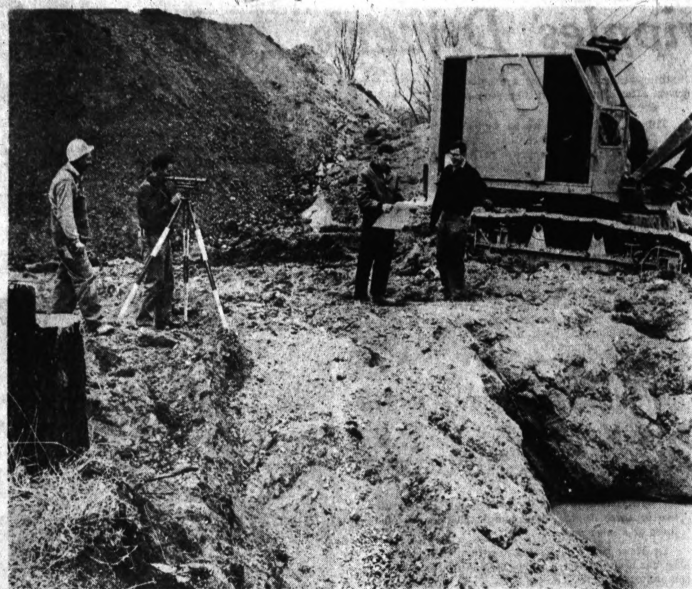
SEWAGE PLANT STARTED — Workers have begun construction of Pontiac's new sewage treatment plant which involves expansion and modernization of the old plant on 23-mile road, just east of town. Now they are digging the hole for the new
