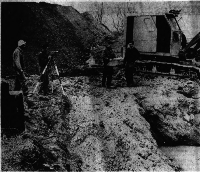
SEWAGE PLANT STARTED —Workmen have begun construction of Romeo's new sewage treatment plant which involves expansion and modernization of the old plant on 32-mile road, just east of town. Now they are digging the hole for the new
