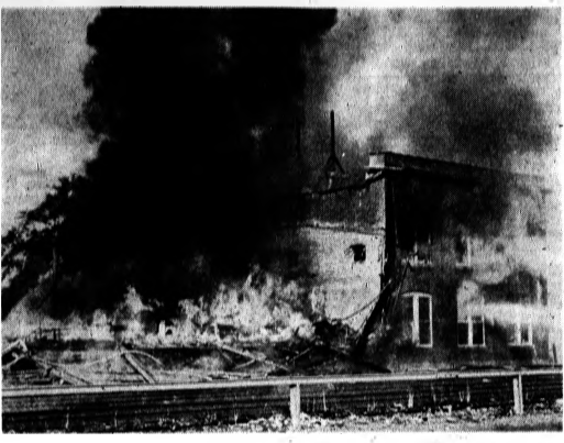
Smoke And Fire Rise From Grand Trunk Warehouse
