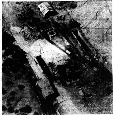
SCENE OF MINE TRAGEDY — An aerial photograph shows two entrances to a coal mine near Barroteran, Mexico, where a searing methane gas explosion trapped 151 to 155 miners two days. It was generally believed all were dead. Before dawn today 23 bodies had been recovered. Seven experts of the U.S. Bureau of Mines in Washington are to reach the small-mining town later today to advise Mexican authorities on faster removal of the dead and restoration of the shattered mine.
