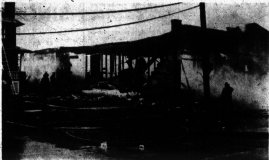
SWEPT BY FIRE —A flash fire and explosions swept through this Royal Oak wholesale plumbing store Saturday morning, causing an estimated $150,000 damage. The Nelson Plumbing Co. store (right), at 332 E. Lincoln, was virtually destroyed.
