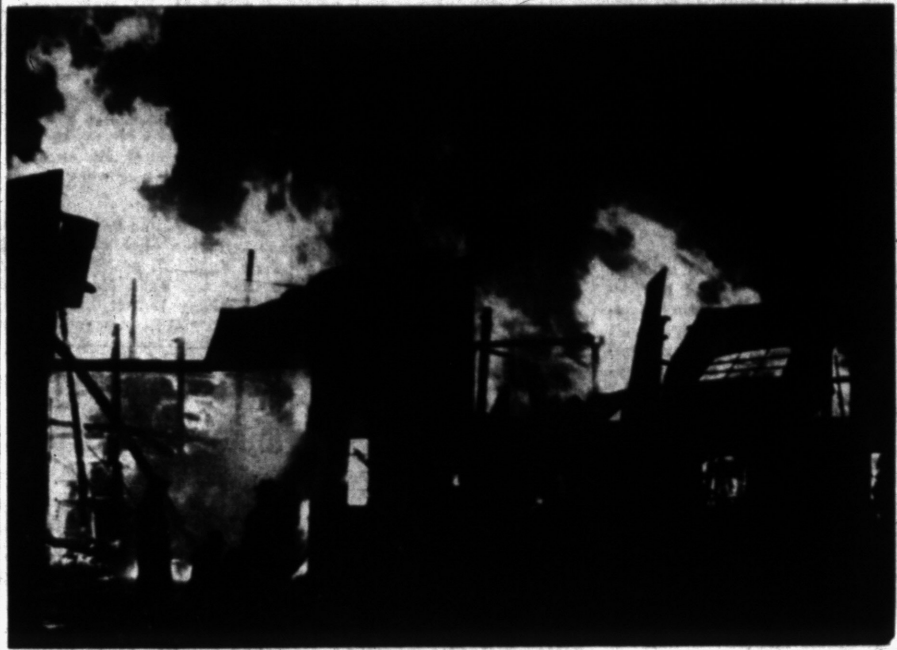
ROOF COLLAPSES—Picture taken above shows building Saturday night, after the roof had fallen. The building was filled with finished lumber.
