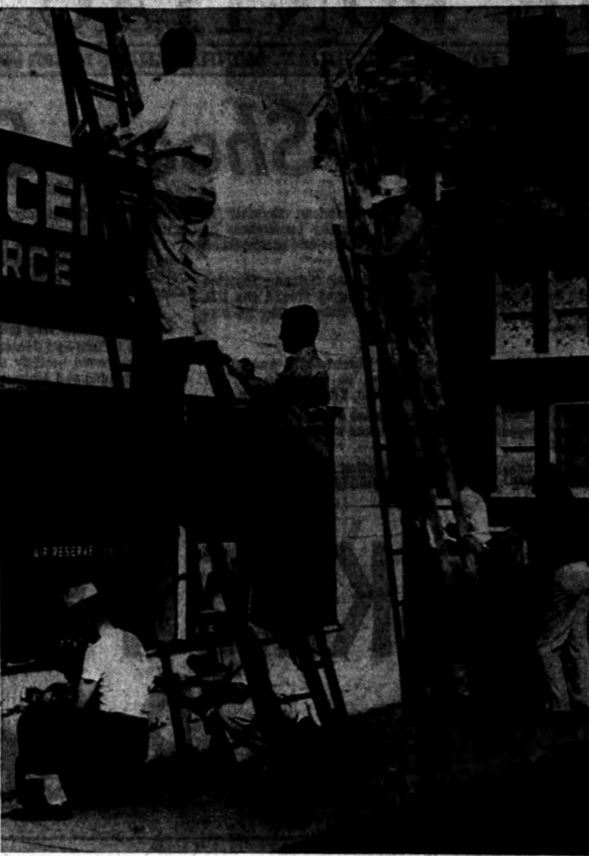
CENTER GETS FIRST FACE LIFTING — Members of the Pontiac Air Reserve Squadron turned out Saturday to give the Air Reserve Center a face lifting. The building which has housed the local air reserve for only a year was cleaned up and given a fresh coat of white paint. With 15 men on the job, according to a squadron spokesman, the building was completed in about five hours time.
