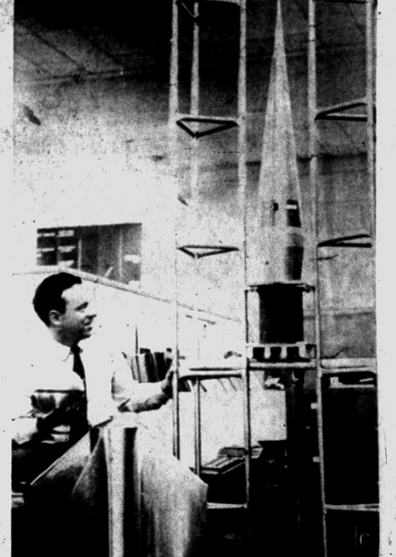
SKY STUDY —Research Engineer Leslie M. Jones of the University of Michigan holds a seven-inch aluminum "sounding sphere" which is carried 400,000 feet into the air by the slender Deacon rocket on the rack and dropped. Both of the devices are part of the university's program of study toward development of an earth satellite. As the sphere falls to earth it radios data on air density and temperature to ground observers.
