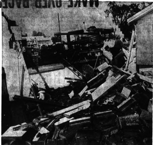
TORNADO DAMAGE — This grocery store in the Williams Crossroads section near Raleigh, N.C., was heavily damaged by a tornado which struck in the Raleigh area yesterday morning. At least six persons were injured by the storm, several at a trailer court. AP Wirephoto
