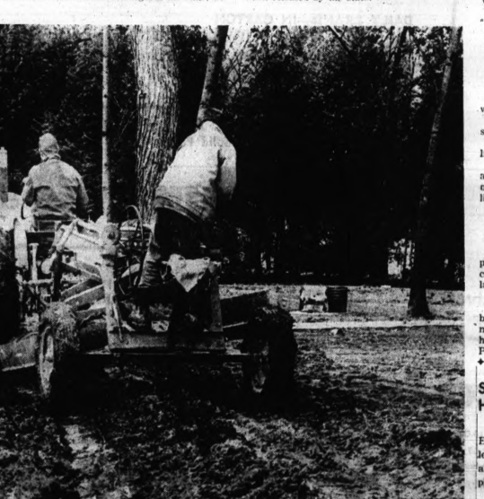
CARVE NEW ROAD — Prisoners from Camp Pontiac work on road construction in one of Oakland County's state parks. Much of the maintenance of Michigan's parks and conservation areas is accomplished through the use of prison labor under supervision of the State Conservation Department. The program, conducted in conjunction with the Michigan Department of Corrections, is believed to be mutually advantageous since it tends to teach prisoners new, honest trades.
