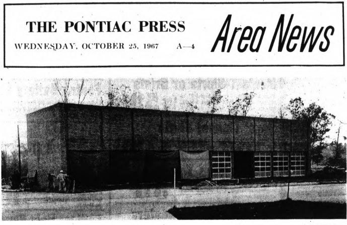
ALMOST COMPLETE—A 10-stall addition to the Bloomfield Township service garage next to the township hall on Telegraph is in the final stages of construction. The $97,000 structure, began last June to be completed by December, will be used to park 10 maintenance vehicles, with a police shooting range and training room on the second level.
