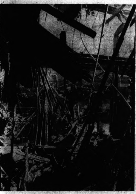
CHARGED REMAINS — Burned debris from the three upper floors lies in pools of water in the gutted lobby of the Roosevelt Hotel. Above, the sun shines through a haze of lingering smoke where the roof collapsed. The section of the building where the lobby was located was hardest hit by yesterday's blaze. (Story, page A-2.)
