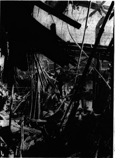
CHARRED REMAINS — Burned debris from the three upper floors lies in pools of water in the gutted lobby of the Roosevelt Hotel. Above, the sun shines through a haze of lingering smoke where the roof collapsed. The section of the building where the lobby was located was hardest hit by yesterday's blaze. (Story, page A-2.)
