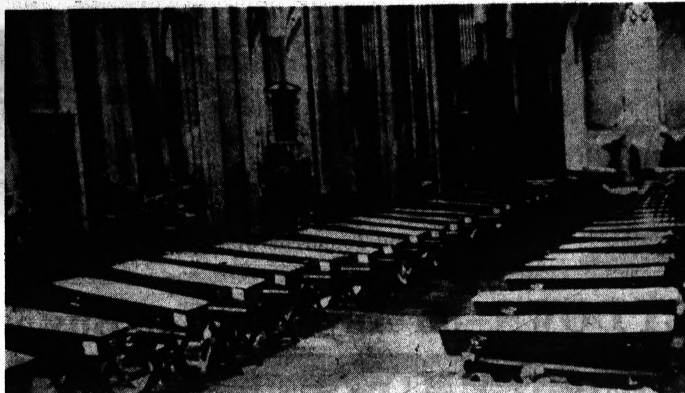
OFFICES OF VICTIMS —Caskets containing the bodies of persons killed in the collision of two passenger trains line the Baur Church at Utrecht, The Netherlands, Tuesday. The crash, in a dense fog between an express train and a commuter train, killed at least 87 persons. It occurred near Woerden.
