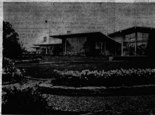
GARDEN ROOM — With the accent on outdoor living, garden rooms such as this one are becoming popular as a means of increasing summertime pleasure. The patio, lawn and flower beds are combined into a functional setting which the glass wall makes a restful extension of the indoor living area.
