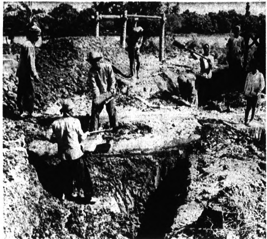
ENTRENCHMENT — These South Vietnamese villagers have been recruited by the government to build an outpost near My Long, in the Mekong Delta. This is part of the "accelerated pacification" campaign which is aimed at bringing as much of the countryside as possible under government control. The digging uncovers remains of previous attempts to establish outposts on the site.
