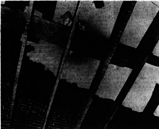
Tornadic Winds Opened the Chapman Hotel Roof
