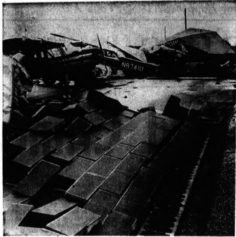
TWISTER DAMAGE — This is the scene at Monroe, Wis., Municipal Airport after a tornado struck early yesterday, causing $86,000 damage to a hangar and seriously damaging several airplanes. No persons were injured.
