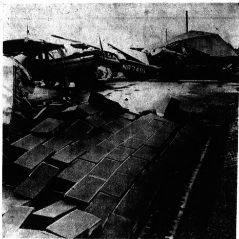
AP Wirephoto TWISTER DAMAGE — This is the scene at Monroe, Wis., Municipal Airport after a tornado struck early yesterday, causing $66,000 damage to a hangar and seriously damaging several airplanes. No persons were injured.
