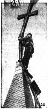
HIGH-LEVEL-WORK — A steeplejack lifts a heavy cross off its pin atop the steeple of Stoughton, Mass., church. The cross, to be refinished, was 140 feet above ground.
