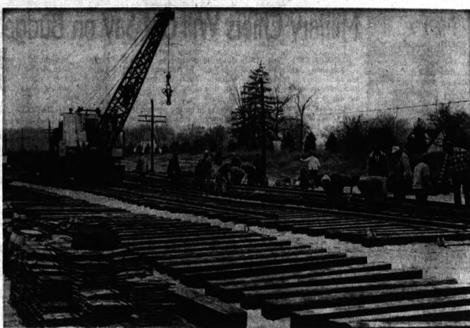
WORKING ON THE RAILS — Piece by piece, nail by nail and day by day, new tracks are laid by workmen for the Grand Trunk Western Railroad at the company's belt yard near Walton and Baldwin. A crane takes some of the heavy work off the shoulders of the construction crew.
