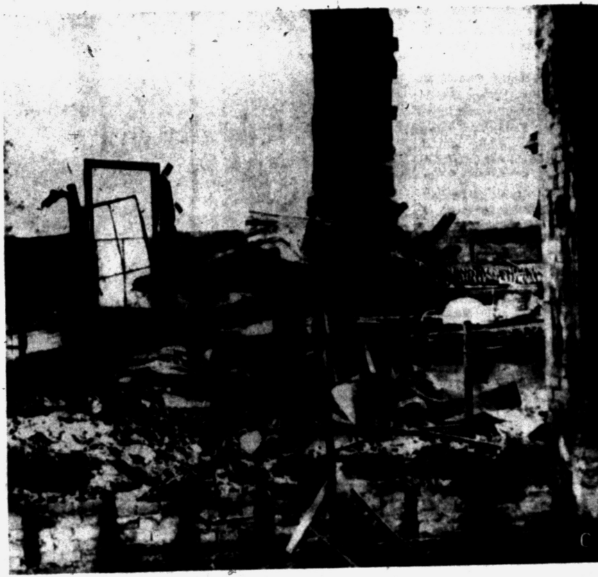
COLLEGE BUILDING GUTTED — Officials at Olivet College went into an emergency session today even as the scorched ruins of the school's administration building, Shipperd Hall, still smoldered. Damage from the blaze was pegged at $800,000. Two other fires, in Michigan's Upper Peninsula, caused another $250,000 damage each.
