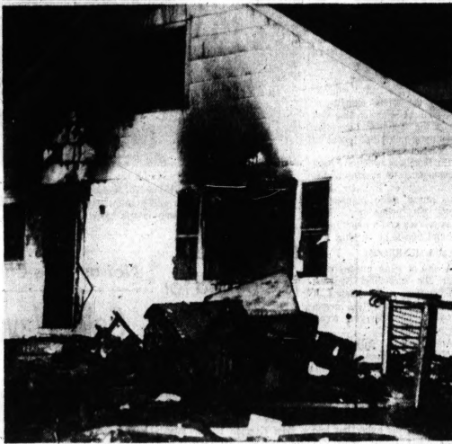
CHARRED RUIN — This is the aftermath of the fire which engulfed the Elbert Cox home in Warren, killing six of nine children. Mrs. Cox is in critical condition.
