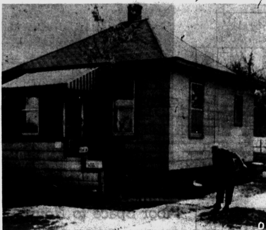
BEFORE — Workmen are beginning the job of building an addition to the Samuel Ashley home on Inglewood. The family had only two small bedrooms and needed more room. They also wanted a garage that they could use as a recreation room.
