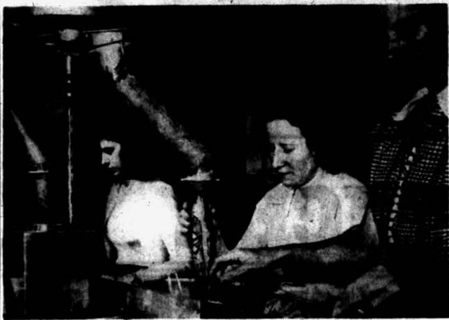
PACKAGING RETAIL BAGS — Girls oversee the filling of the clear plastic bags that are a familiar sight on your grocer's shelves. Afterwards the bags are weighed and heat sealed mechanically.
