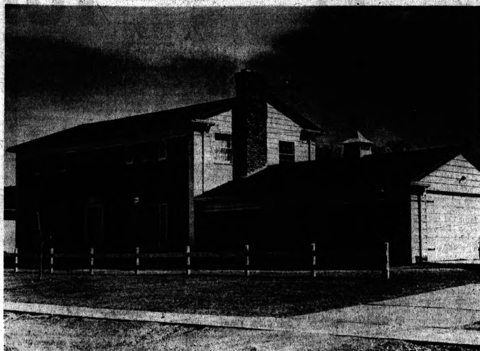
IN WATKINS HILLS — This was a model home for the subdivision. Last December the Roy Shadrick family moved into the two-story brick and frame house. Ward Ross was the
