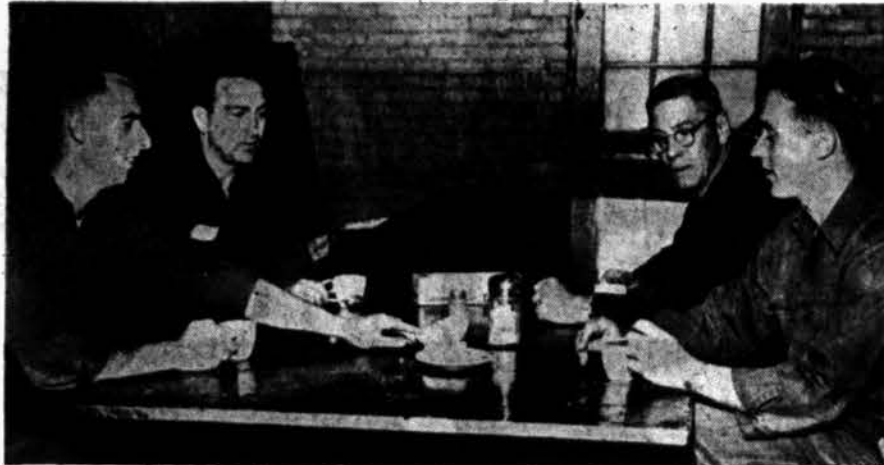
THE COFFEE BREAK — No fire alarm spoiled their coffee break this time. Firemen enjoying a moment of leisure are (lower left) Jim Booth, (upper left) Bernie Martin, (upper right) William Breakey and (lower right) Larry Melrose. Coffee's always on at the fire hall.
