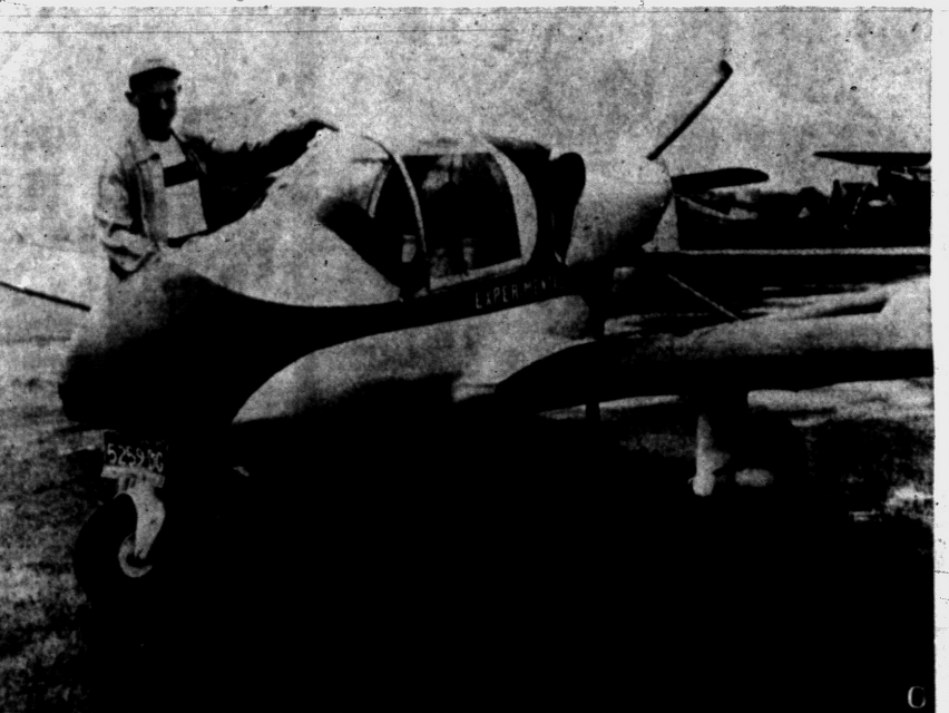
NOW IT'S A PLANE — With the wings unfolded, Bryan's Auto-Plane is ready for the air. The builders claim a cruising speed of from 85 to 90 miles an hour, with a flying range of about 400 miles without taking on additional fuel.
