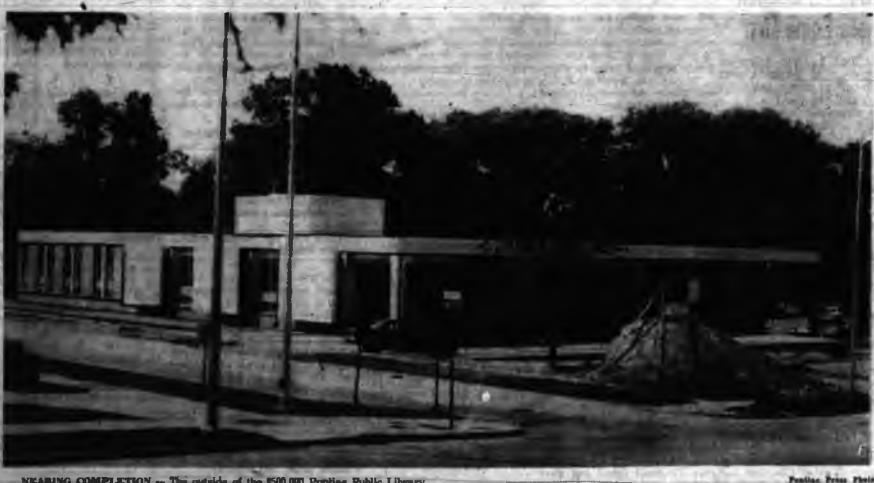
NEARING COMPLETION — The outside of the $500,000 Pontiac Public Library building is finished as its September opening date approaches. It'll take about two weeks to move books into Pontiac's newest public building and it is turned over to the city Sept. 15. The library fronts on Pike street (right) and sides on Park street (left) in the Civic Center.
