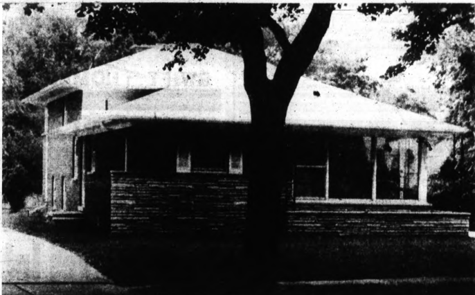
ON A NARROW LOT — This tri-level brick home is built on a 50-foot lot on West Iroquois road. Owners, the Leonard Sundahls, used a stock plan, had Frericks Brothers do the building. Stone
