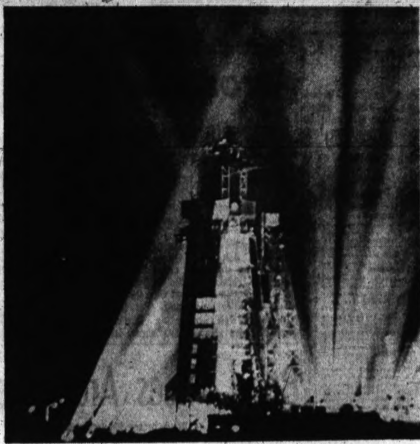
ATLAS ON PAD — The Atlas missile which boosted Astronaut John Glenn into space today stands on its pad early this morning as workmen make last minute preparations. The missile is surrounded by a service gantry.
