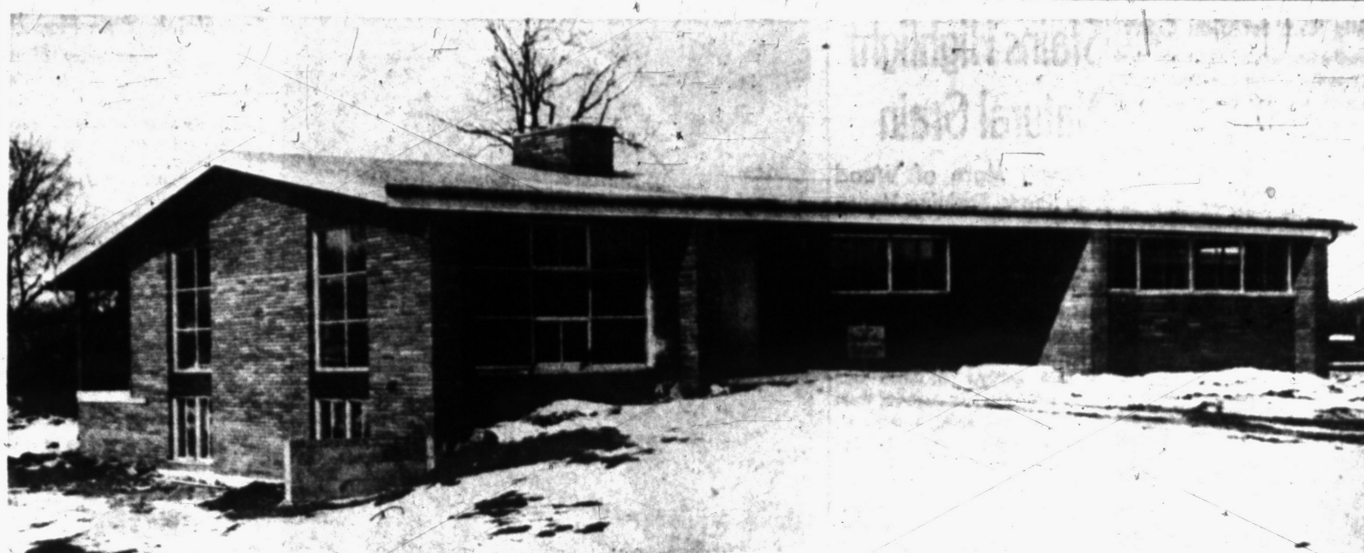
CALIFORNIA CONTEMPORARY—Open to the public in Lone Pine Village Sun-Homes Inc. Though designed for Michigan winters, the spaciousness of the California day will be this distinctive contemporary-type home, at 4774 Keithdale by Style-Rite style structure contributes to a feeling of true outdoor living all year long.
