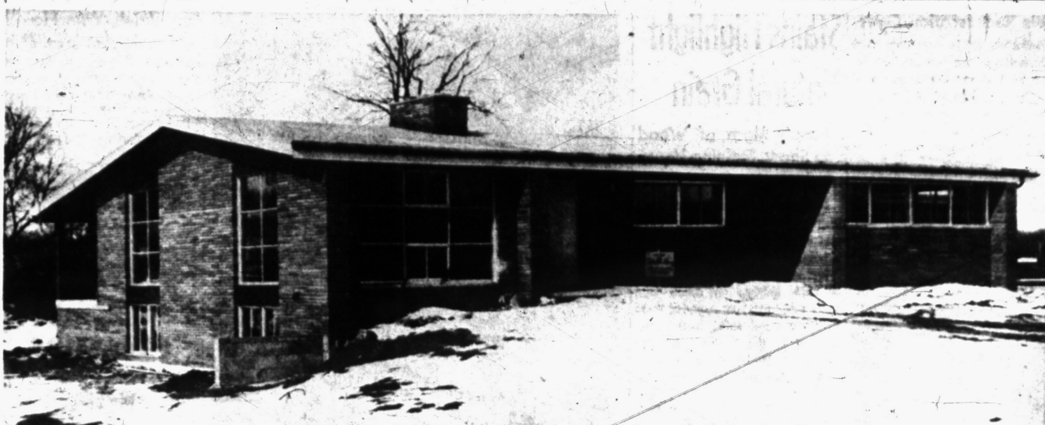
CALIFORNIA CONTEMPORARY—Open to the public in Lone Pine Village Sun-Homes Inc. Though designed for Michigan winters, the spaciousness of the California-style structure contributes to a feeling of true outdoor living all year long.
