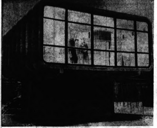
SOVIET SHOWCASE — Resembling a modernistic television set, the first house to be made of plastic materials nears completion in Leningrad, U.S.S.R. The boxlike dwelling is heated with the help of hot-air fans. Photo and caption from official Soviet source.
