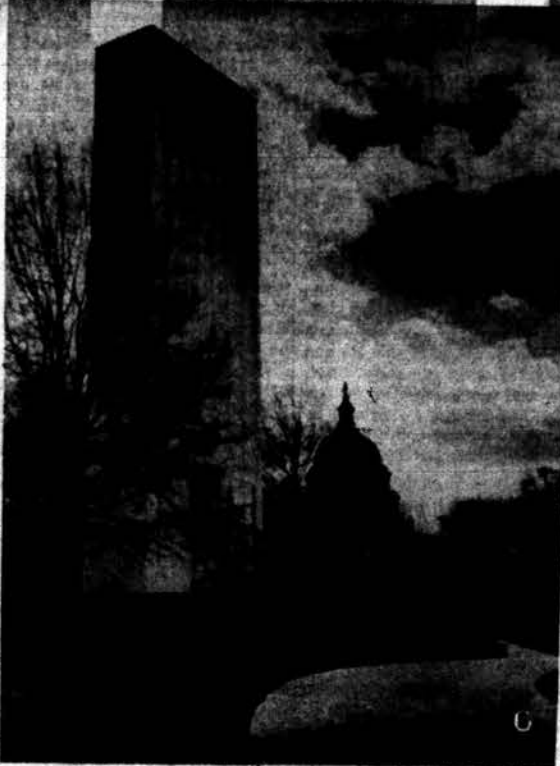
TAFT MEMORIAL — Workmen put the final touches on the slim 100-foot pink marble bell tower — a memorial to the late Sen. Robert A. Taft of Ohio — near the U. S. Capitol building. The new monument will be formally dedicated April 14. See story on Page 60.
