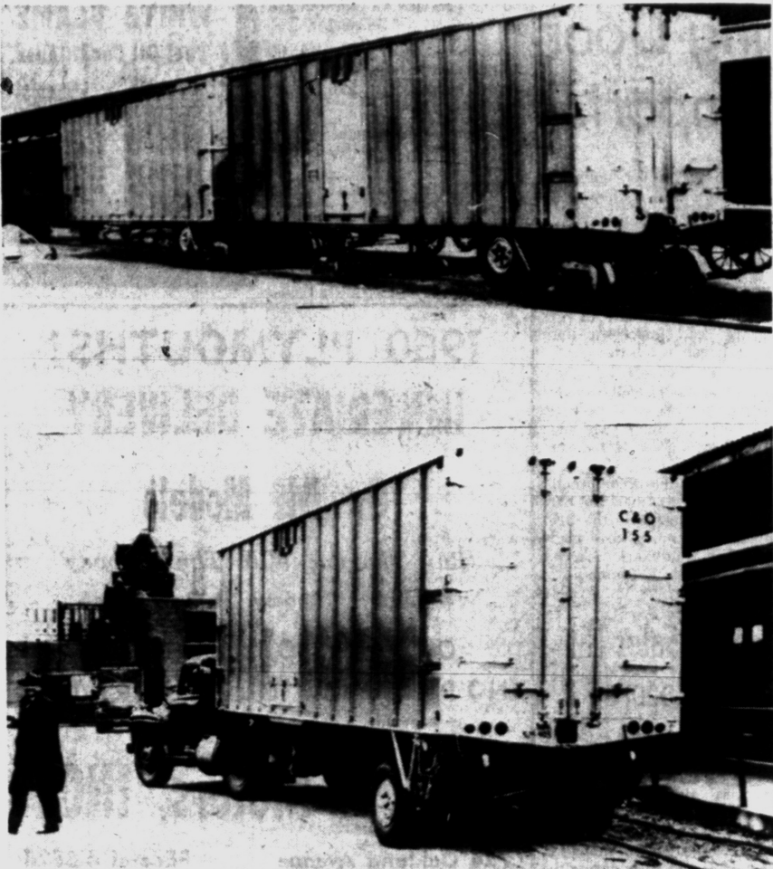
TO TRAVEL IN MICHIGAN — Freight cars equipped with dual tires and flanged wheels on railroad tracks (top) are hauled to destination (below) during inauguration this week of railvan service by C & O Railway between Grand Rapids and Detroit. The truck-trailer vehicles operate with equal ease on rails or highways. Each van is 26 feet long and has a load capacity of 25,500 pounds.
