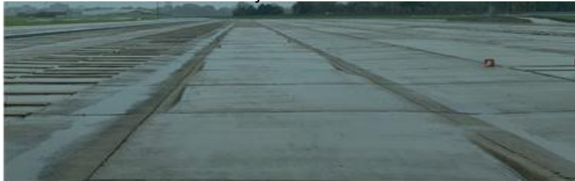
Figure 5.9: controlled proving ground test tracks used to generate deterministic vehicle dynamics disturbances for ground truth labeling
