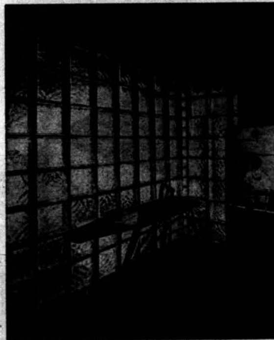
BRIGHTEN UTILITY ROOM — Large panels of glass block "borrow" daylight from the kitchen for the utility room in this modern home. In addition to the functional purpose of brightening the utility room which has no direct source of daylight, the shining glass block panels add to the attractiveness of both rooms. Impervious to moisture or condensation, the panels can be cleaned simply by wiping with a damp cloth.
