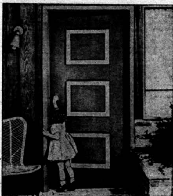
DRESSED UP STEEL doors open in home building this year. Light enough for child to open, doors eliminate shrinking, warping and swelling caused by heat and moisture extremes. Designs match any home style.
