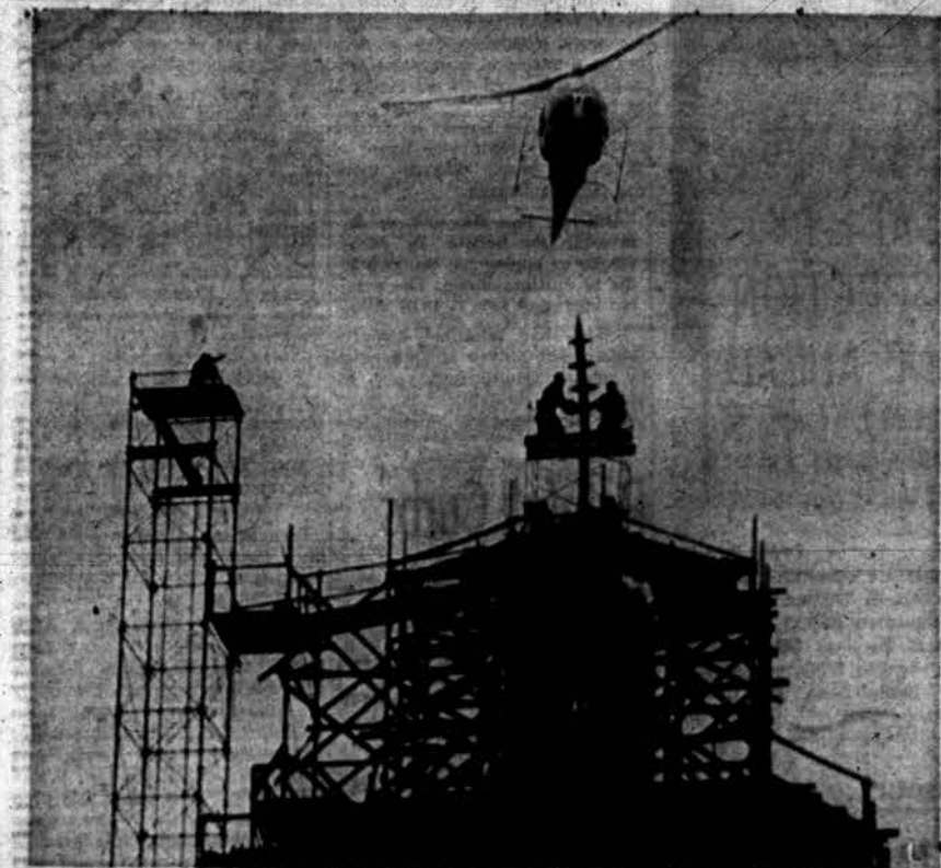
SPIRE FROM THE SKY — A helicopter holds the third of five spire sections steady while workmen fasten it in place on top of the Kirk-in-the-Hills Church tower, 150 feet above ground. The unique use of the whirlybird in high construction projects succeeded this morning after a previous attempt last week failed.
