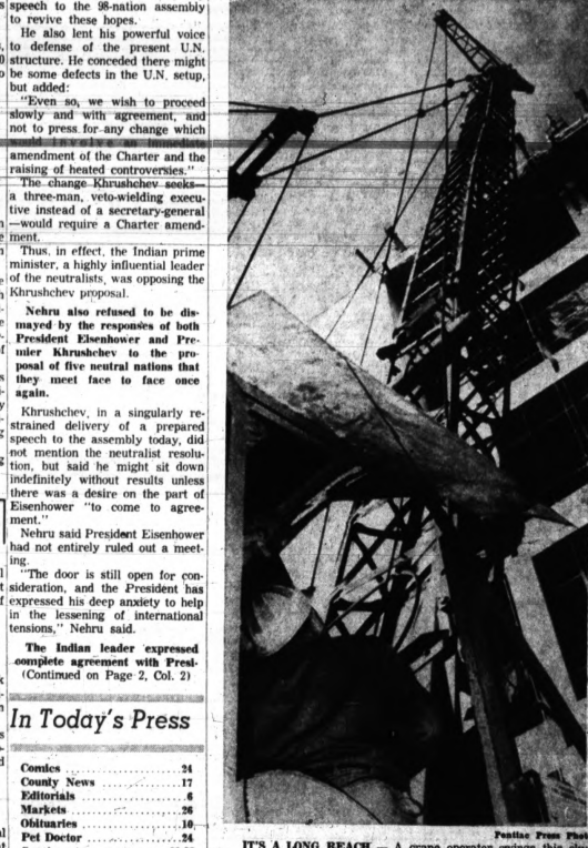
IT'S A LONG REACH — A crane operator swings this skyscraper high crane along the west side of the new county courthouse in the County Service Center, lifting large slabs of marble to workmen on scaffolding above. Crews are racing the calendar in hopes of having the six-story structure enclosed before the cold weather arrives. The building is expected to be completed next summer.
