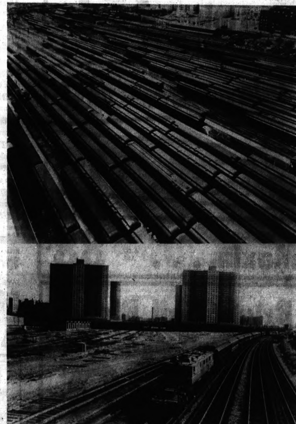
BIG DIFFERENCE — In 1961, the Mott Haven passenger yards in New York City were jammed with passenger trains (top photo). Today the yards are almost empty and apartment houses cover some of the old tracks.
