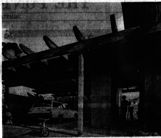
CAR HOUSING —Striking shelter for the family coach is this carport with its excitingly designed roof structure. Heavy, rough-sawn Douglas fir beams are stained chocolate as contrast to aquamarine siding. Full height
