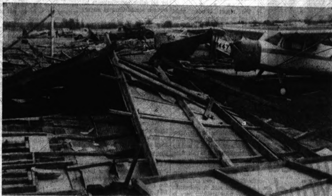
HANGAR WRECKED — A section of debris marks the spot at Young Airport near Ann Arbor where winds took over control yesterday. Seven airplanes were damaged when the
