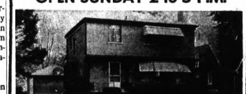
HELLO — Adding screens and a low porch deck resulted in this distinguished entrance area. Screens are spaced Douglas fir 2x4s in a framework of 2x4s. They're screwed over existing bevel siding on either side of door; projecting sections give privacy to an adjacent window. Deck of fir 2x4s on edge raises porch to door sill level.
