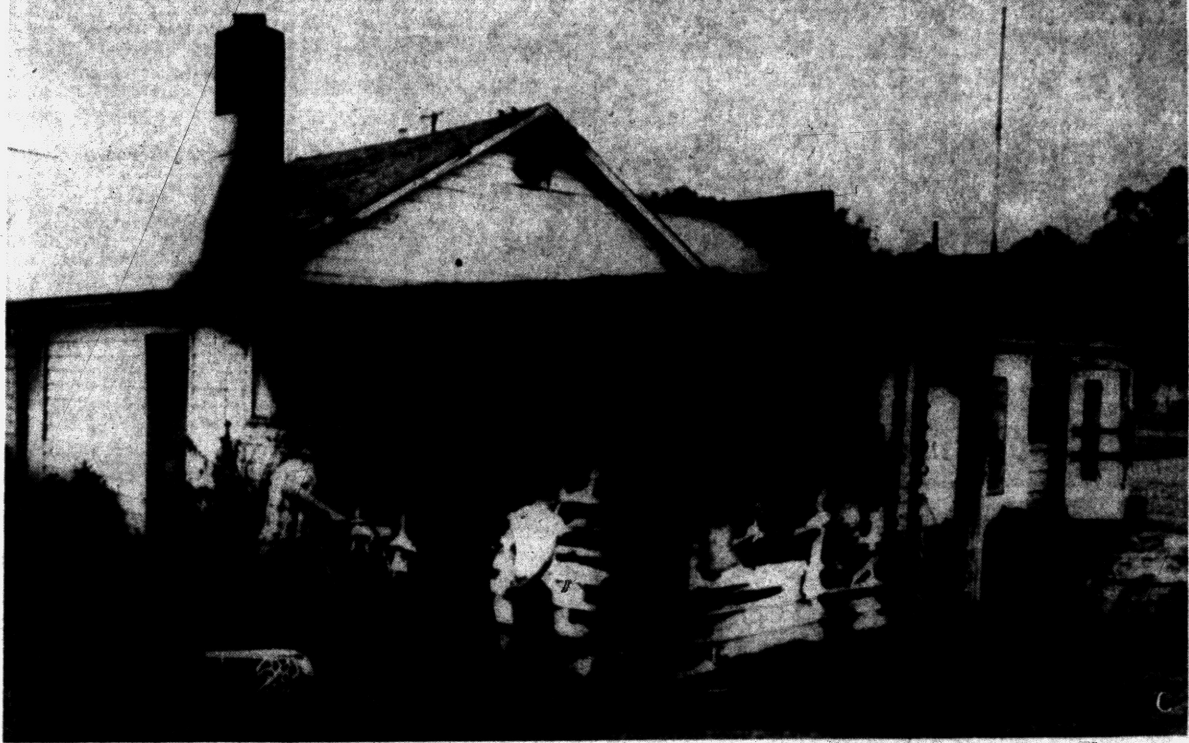
SCENE OF TORCH BURNING? — These are the charred sections of the Latreille Dry Cleaners on Davison Road, Flint, and the S. & S. Grill next door, burned Sunday night. Investigators today believe there may be a connection between this fire and the burning of teamster official Frank Kierdorf.
