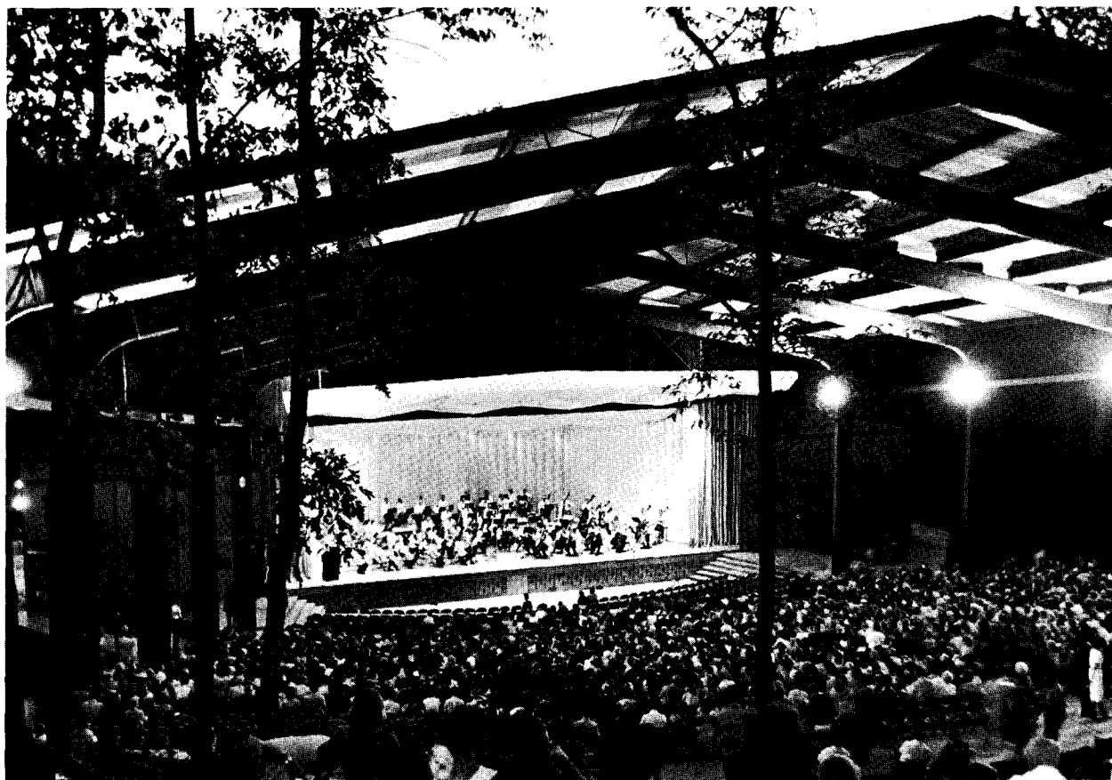
HOWARD C. BALDWIN MEMORIAL PAVILION, designed by O'Dell, Hewlett & Luckenbach Associates, provides 2,138 sheltered seats, with room for an equal number of people on the grass in the natural amphitheater around it. The fiberglass structure on the stage—the LULA C. WILSON MEMORIAL CONCERT SHELL—incorporates a flexible ceiling that can be adjusted to balance the sound. It was designed by Christopher Jaffe, noted acoustical expert.
