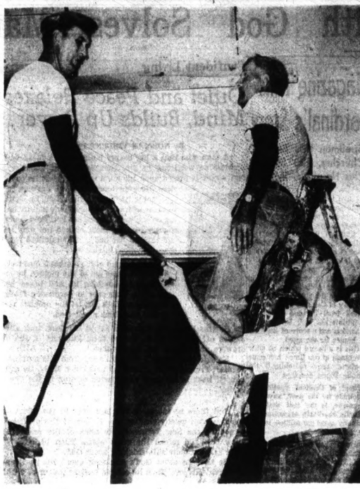
BRACING CEILING — Edsel Malkin of 1374 Joslyn Rd., from left, Lawrence Ferman of 1614 Opdyke Rd. and Peter Vanderhook of 94 E. Beverly St. brace the ceiling in preparation
