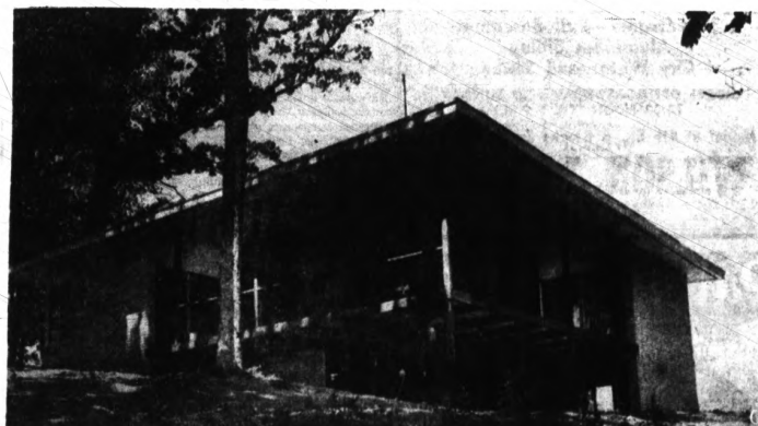
CANTILEVER CONSTRUCTION —The Ward Veen house at Lake Sherwood is cantilevered over the hillside. A combination of gray Roman brick and redwood, the house has six rooms on
