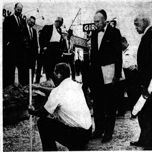
HOW HIGH THE ROAD — Circuit Judge Clark J. Adams (second from right) yesterday visited Union Lake to view the difference in level between old Union Lake Road and the new roadway under construction, the issue in a court dispute between local businessmen and the County Road Commission. Measuring is
