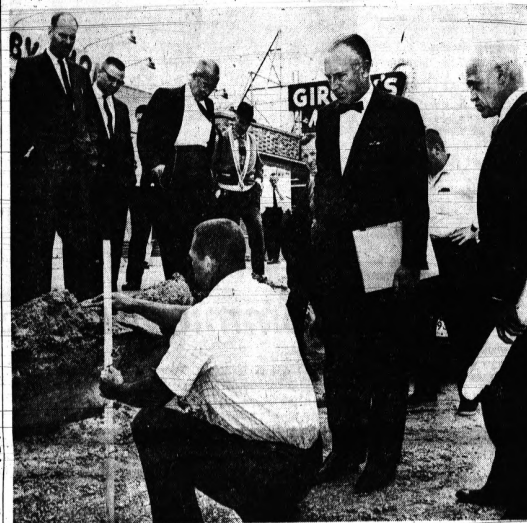
HOW HIGH THE ROAD — Circuit Judge Clark J. Adams (second from right) yesterday visited Union Lake to view the difference in level between old Union Lake Road and the new roadway under construction. The issue in a court dispute between local businessmen and the County Road Commission. Measuring is road commission engineer David Burns, while Nerec Alax (right), engineer for the businessmen, looks on. Businessmen claim the planned new level of two feet lower will be unsafe for the public and harmful to them. Judge Adams set 9 a. m. tomorrow for a hearing on continuing an injunction that has halted construction.
