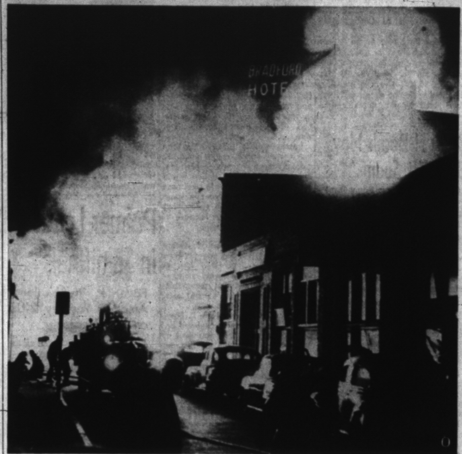
FIRE FLARES IN FILM SHOP —Firemen battle multiple-alarm blaze in the city in a week, the fire started in a film shop, wrecking several film equipment offices and driving 10 families from their homes.
