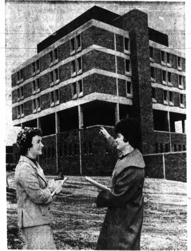
Construction on the new Rochester Suburban Unit of Crittenton General Hospital is moving right along due partly to the efforts of the Rochester Women's Club which has so far donated $10,000 to the building fund. Club members checking on the building progress are from left, Mrs. Kenneth Hock and Mrs. William Keinath, both of Rochester.
