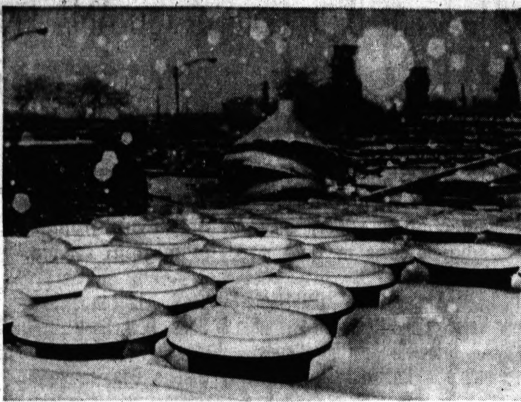
WEIRD CHICAGO SNOW SCENE —An otherworldly effect is produced as snowflakes drift down on a construction site in downtown Chicago yesterday. The rows of mustroom-
