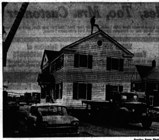
MOVING DAY — At 11:45 a. m. yesterday this four-family house, owned by the National Bank of Detroit, began to move slowly up Walnut Street toward the center of Rochester. An hour and a half later, after traveling along West University to Main and north on Main to Woodward Street, the stately 50-ton dwelling was parked securely at its new location. The house, moved by Goetz House Moving Co., Warren, is at 333 Woodward St., site of the former home of Mrs. Cora Barwick which was partially destroyed by fire New Year's Day, 1959.
