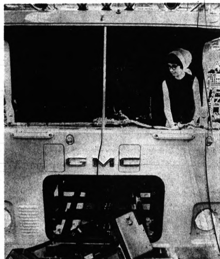
Wiring, Insulation, Instrumentation Are Installed
