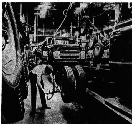
Pneumatic Wrenches Are Used For Wheel Installation
