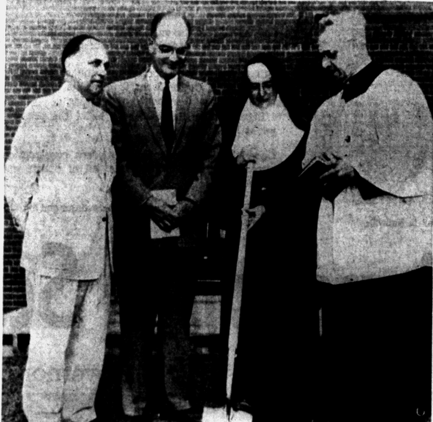
START CONSTRUCTION — Taking the first shovel to begin construction of a $650,000 powerhouse and laundry building at St. Joseph Mercy Hospital yesterday was Sister Mary William, hospital administrator. Others participating in the brief ceremony were (left to right) Dr. Robert J. Mason, president-elect of the hospital staff; Dr. Robert R. Wessels, president; and Father Michael O'Reilly, of St. Michael's parish.
