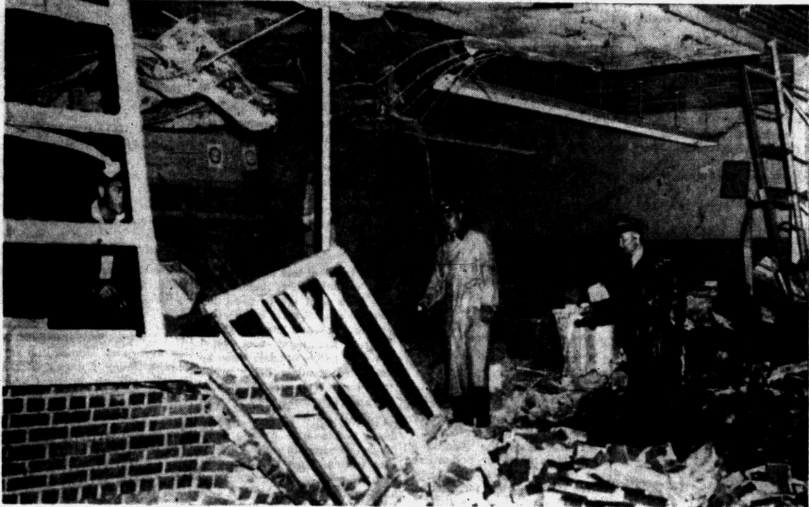
BLASTED SCHOOL — Police examine wreckage of wing at newly desegregated Hattie Cotton school in Nashville
