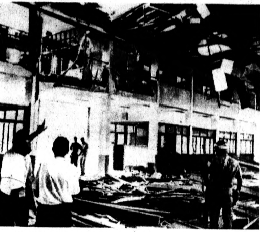
HIT BY BOMB — Debris dangles from the roof and litters the floor at the main entrance of the civilian terminal at the Saigon airport after a terrorist bomb exploded today. More than 40 persons were injured as every window in the building was blown out and a section of the roof blown down.
