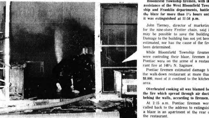
APPLIANCE STORE BLAZE — Bloomfield Township firemen battle a blaze which gutted the interior of Fretter's Appliance Store, 1650 S. Telegraph, last night. Merchandise valued at more than $100,000 was destroyed.
