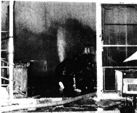
APPLIANCE STORE BLAZE — Bloomfield Township firemen battle a blaze which gutted the interior of Fretter's Appliance Store, 1650 S. Telegraph, last night. Merchandise valued at more than $100,000 was destroyed.
